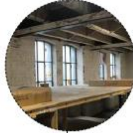
Existing brick facade and windows
