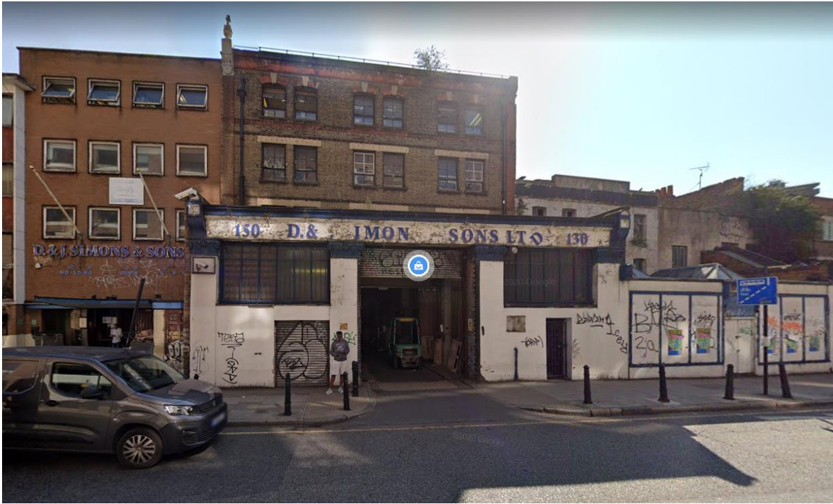
Figure 3 DJ Simons Building, Existing Hackney Road Elevation
