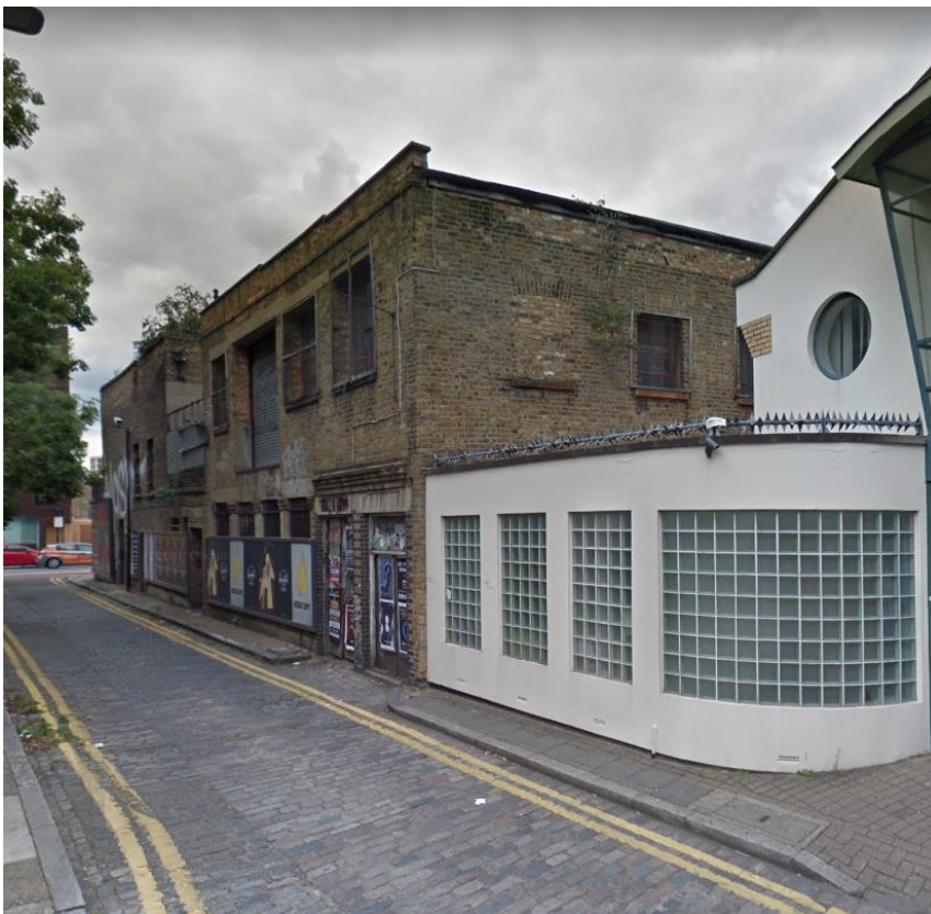
Figure 4 Existing Strouts Place Building Elevation
